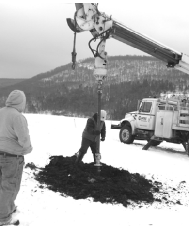
DCEC lineman drilling holes for wells
