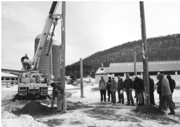
DCEC installing utility poles on SUNY Delhi campus
